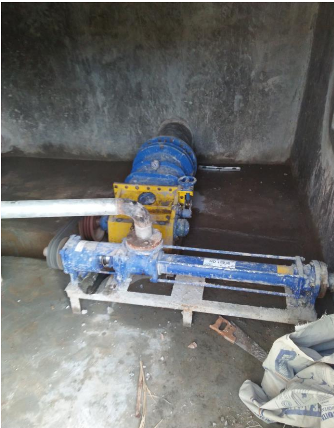
Proposed Pump Type Installation Output 10,000 m 3 /H
